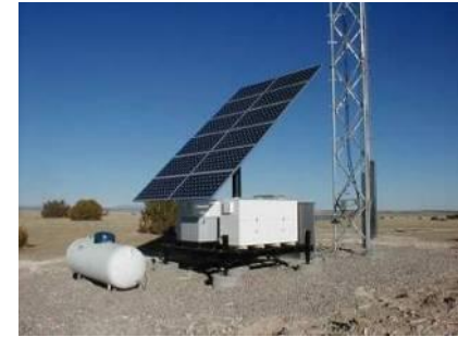
BTS with solar modules
